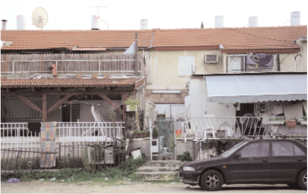
WochenKlausur, Home Improvement Service , 2012. Artist-performed apartment renovations in the Jessy Cohen neighborhood in Holon, Israel, at no cost to residents.
